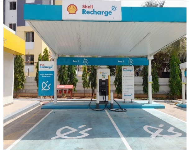
Fig. 2: 3.3 kW AC Chargers for 2-wheelers and 3-wheelers
