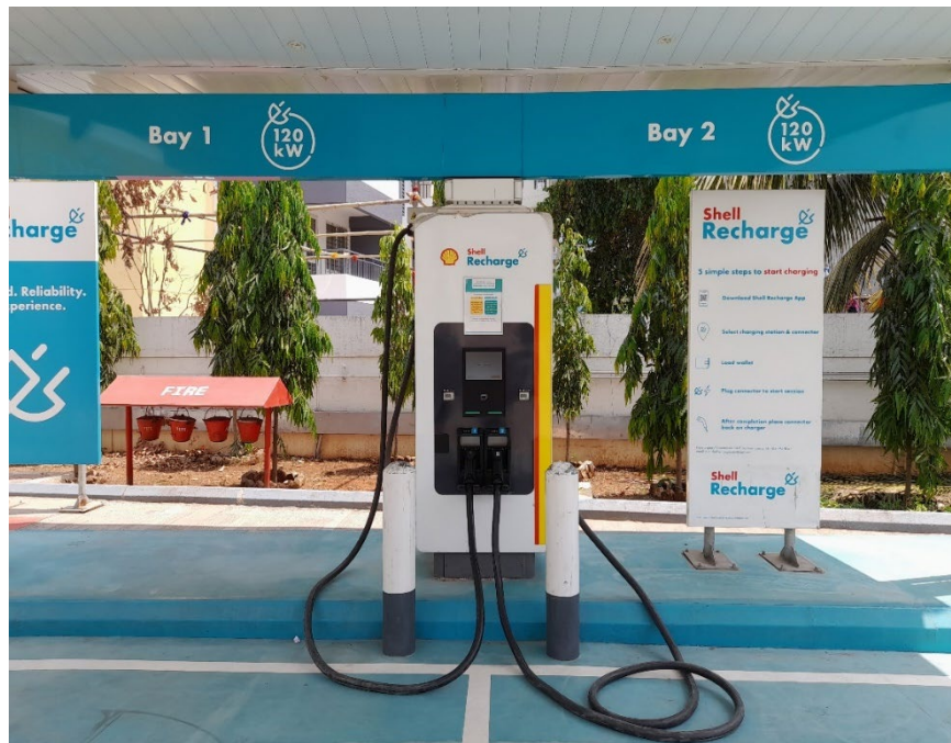
Fig. 3: 120 kW DCFC with 2 CCS 2 ports
