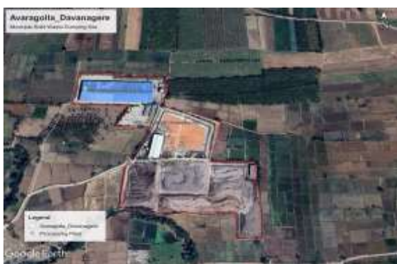
Figure-1(a): Municipal Landfill site, Avaragolla, Davangere
