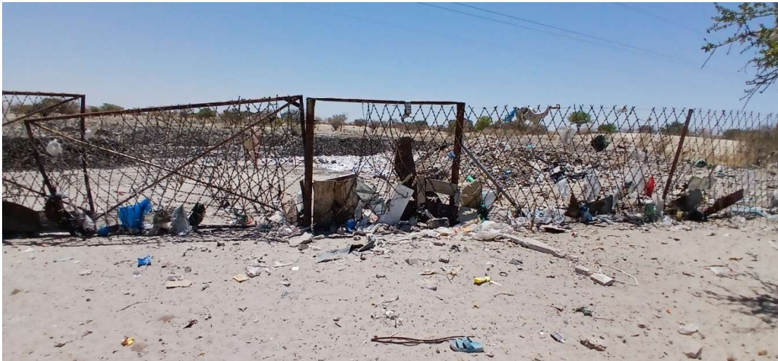
Fig. 15: Fence of the disposal site
